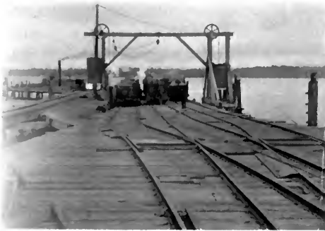
NORTH JETTY APRON WHEN THE CARS ARE HAULED OFF THE BARGE BY A POWERFUL ENGINE AND CABLE.
